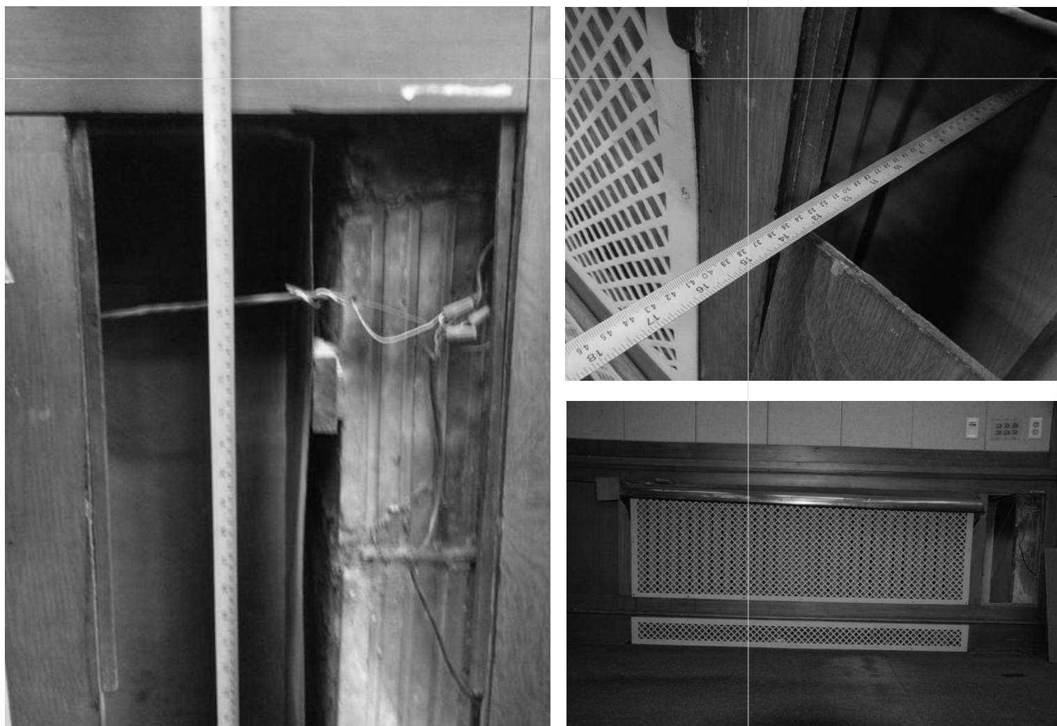
PHOTOGRAPHS OF EXISTING RADIATOR RECESSES AND GRILLES, NORTH ELEVATION.
