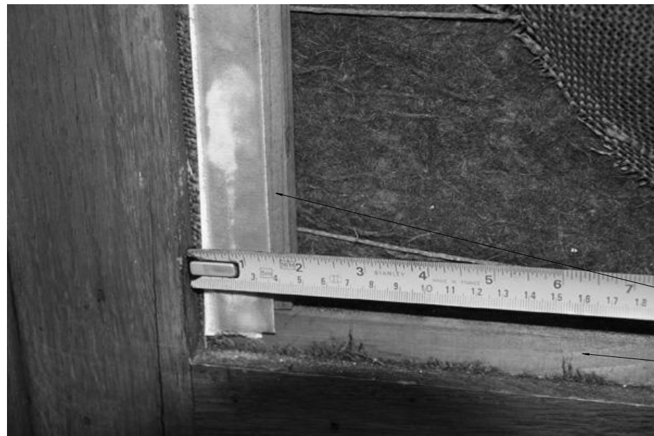
PHOTOGRAPHS OF TYPICAL EXISTING ACOUSTICAL PANEL DETAILS IN ROOM 260 TO BE REMOVED.
